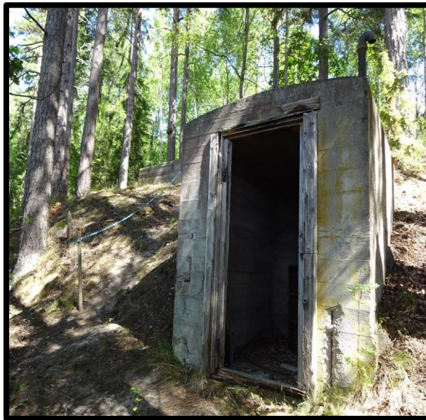
A more intact Water Works Structure
