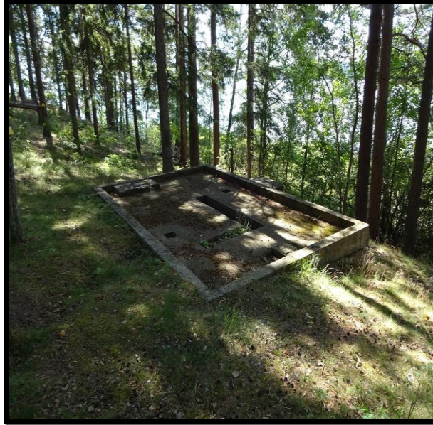
Foundation of the Water Works Building 38
